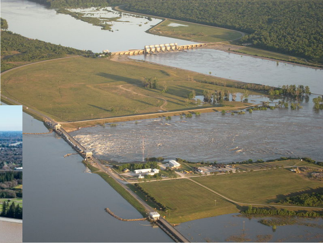
USACE – Mississippi Old River Control Structure Louisiana
