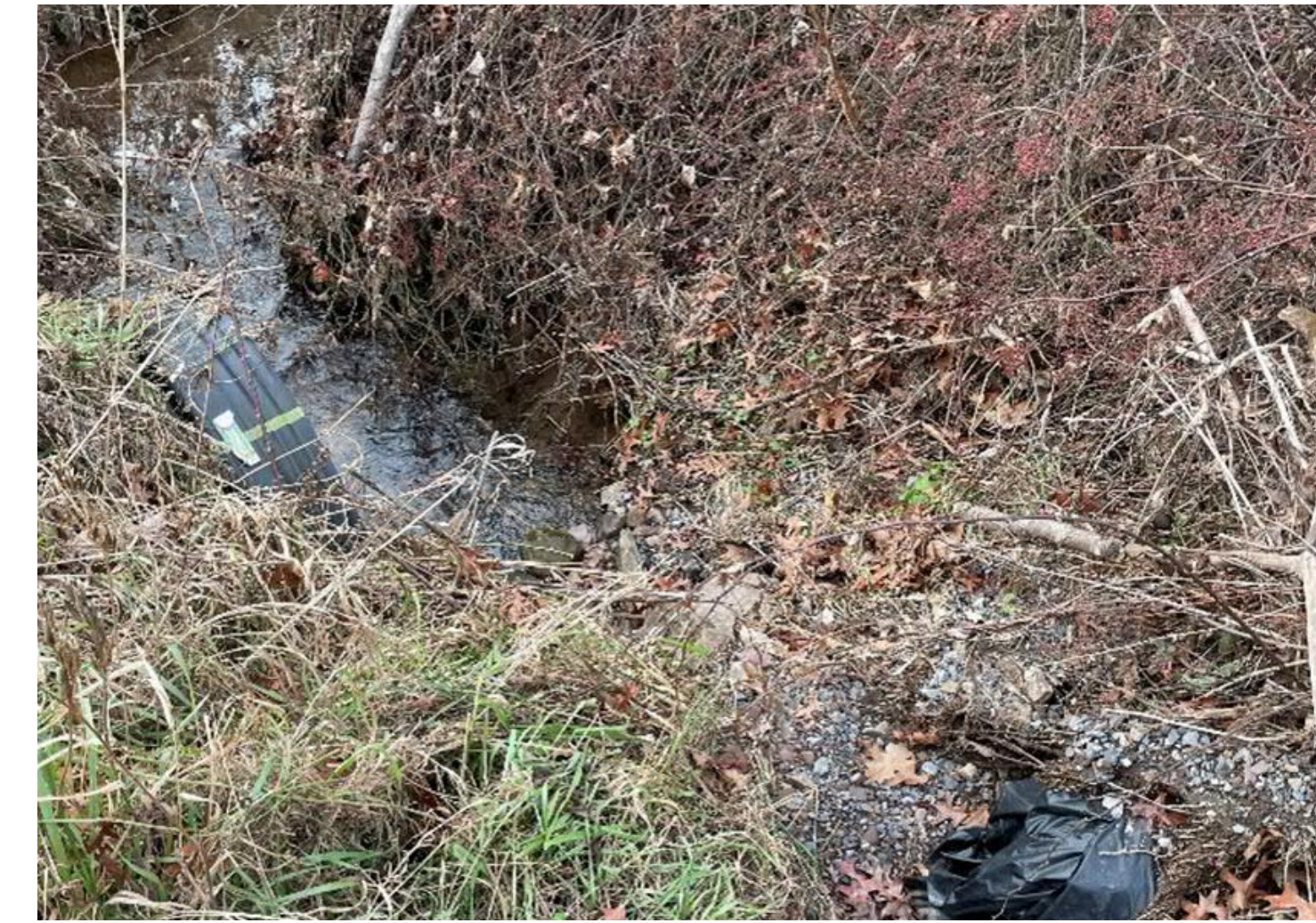
Problems: Flooding/Sedimentation Mitigation Concepts: Culvert Replacement
