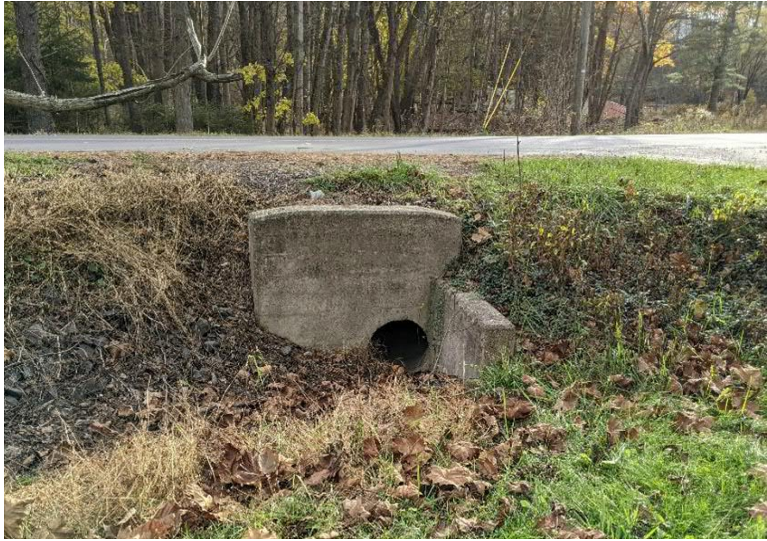
Problems: Flooding/Sedimentation Mitigation Concepts: Culvert Replacement
