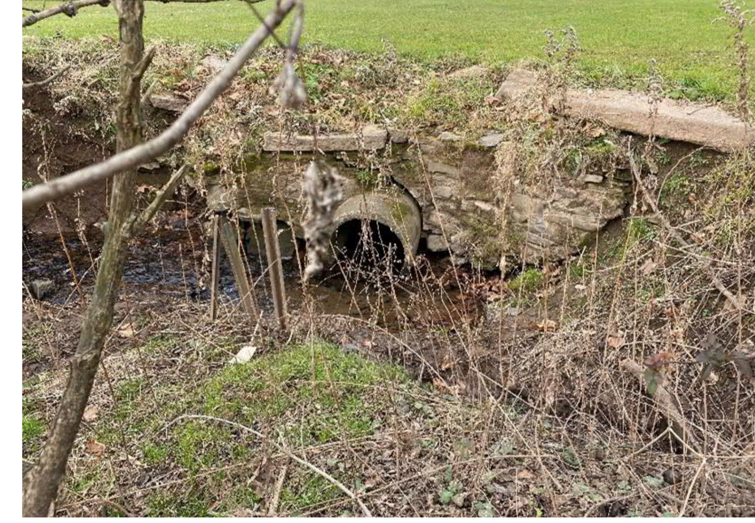
Problems: Flooding/Sedimentation Mitigation Concepts: Culvert Replacement
