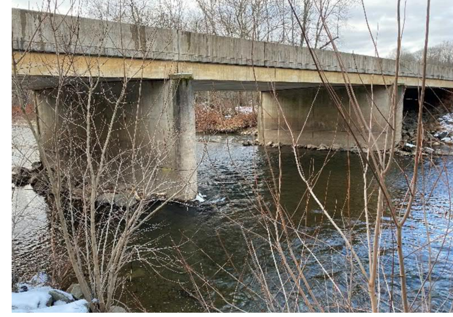
Problems: Erosion/ Flooding / Infrastructure Mitigation Concepts: Pier Scour Protection / Floodplain Reconnection
