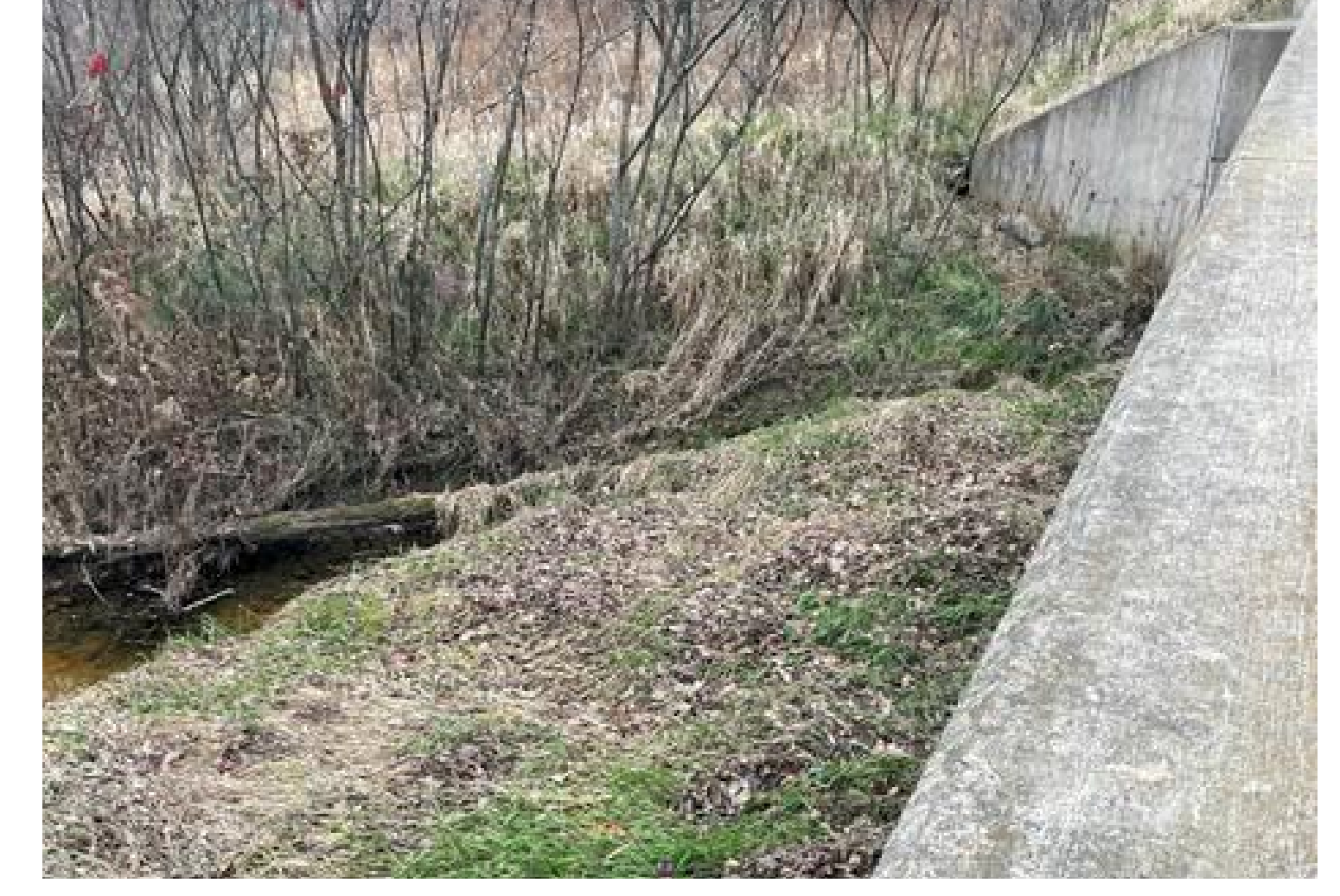
Problems: Flooding/Sedimentation Mitigation Concepts: Bridge Replacement
