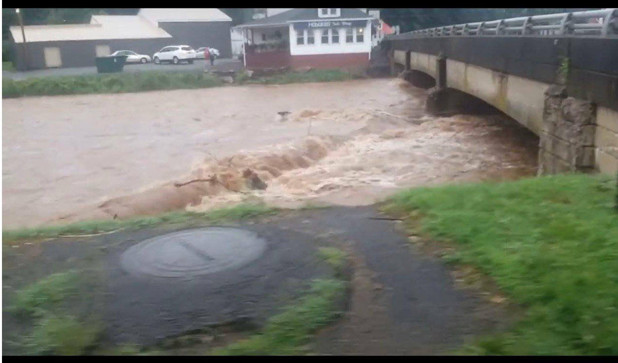
Figure 7.1 July 25, 2018 storm event shows water within Fishing Creek (Benton) just below the bridge low chord. This still shot was taken from a video uploaded to YouTube by a local resident (Redneck News Benton).
