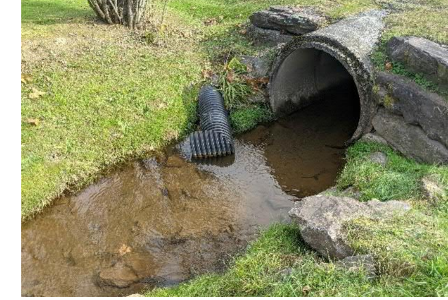
Problems: Flooding/Sedimentation Mitigation Concepts: Culvert Replacements
