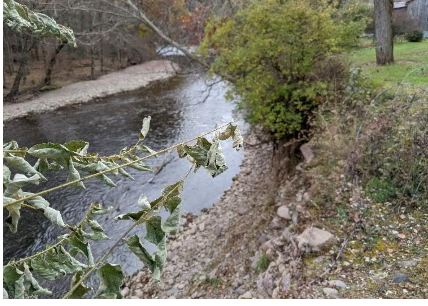
Problems: Erosion/Flooding Mitigation Concepts: Floodplain Reconnection/ Streambank Stabilization
