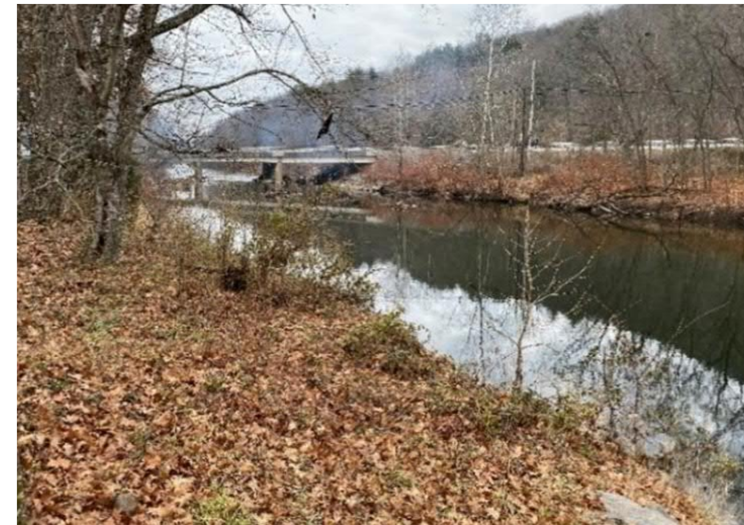
Problems: Flooding/Sedimentation Mitigation Concepts: Structure Removal/ Streambank Stabilization
