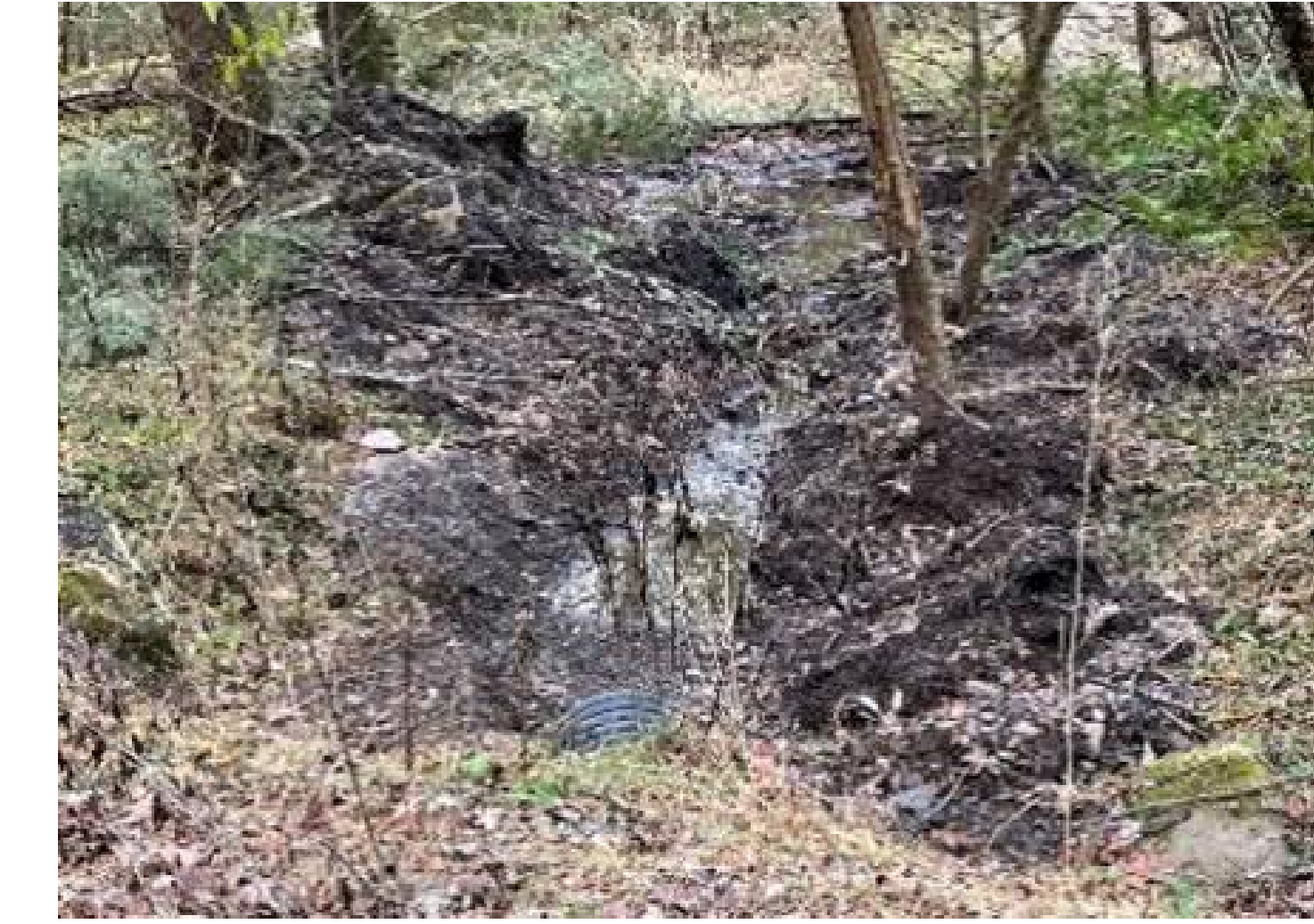
Problems: Flooding Mitigation Concepts: Culvert Replacement
