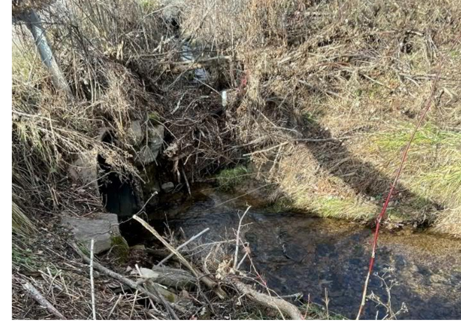
Problems: Flooding/Sedimentation Mitigation Concepts: Culvert Replacement
