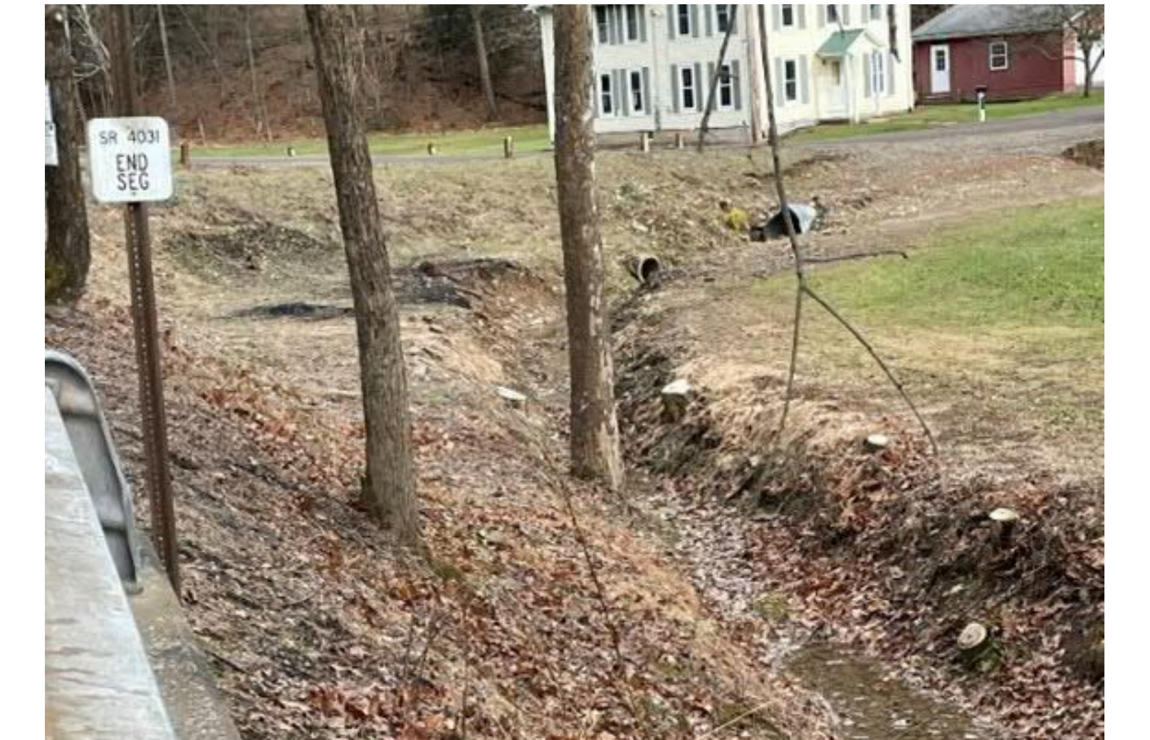
Problems: Flooding/Sedimentation Mitigation Concepts: Culvert Replacement
