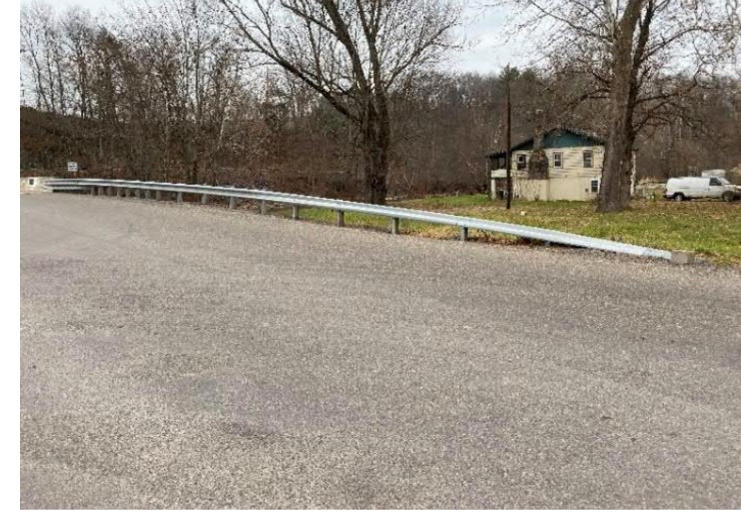
Problems: Flooding Mitigation Concepts: Property Buyout/ Relocation
