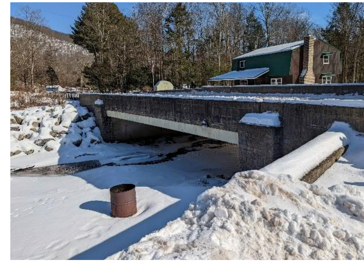
Problems: Flooding/Sedimentation Mitigation Concepts: Culvert Replacement / Bridge Replacement
